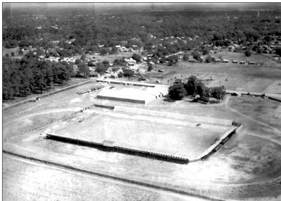
The football stadium formerly located at the Sumter fairgrounds is seen.
