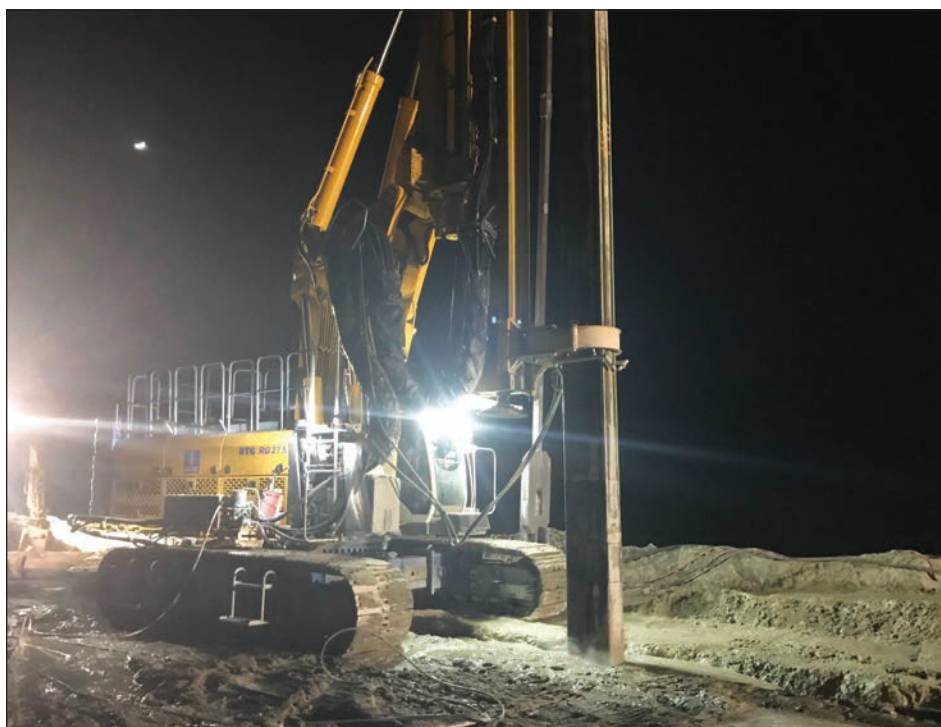
Special to the Lake Okeechobee News/USACE/Torres LAKE OKEECHOBEE – Work on a cutoff wall in the Herbert Hoover Dike continues round-the-clock.
