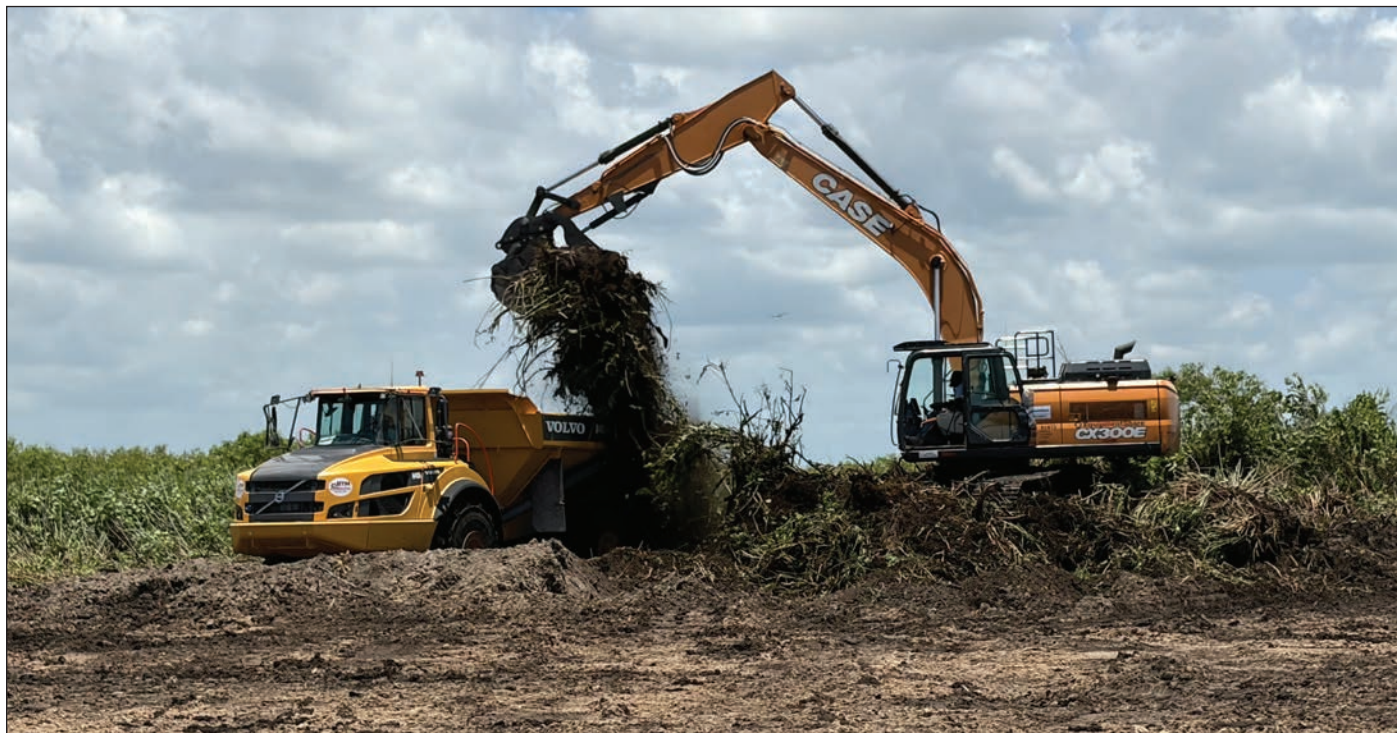
BUCKHEAD RIDGE -- Taking advantage of low lake conditions, Florida Fish and Wildlife Conservation Commission contractors Texas Aquatics are scraping muck and vegetation from 287 acres of the bottom of Lake Okeechobee near Buckhead Ridge. The muck and dead vegetation is being trucked to a spoil site outside the dike. [Photo by Katrina Elsken/Lake Okeechobee News]
